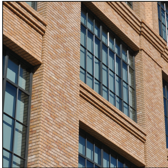
BRICK VENEER CLADDING ON CAST STONE PANELS
